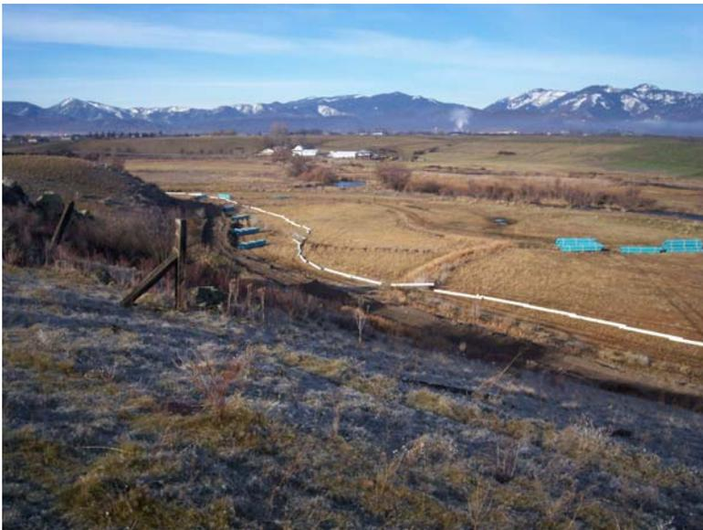
*Installation of pipeline to replace earthen ditches.*
