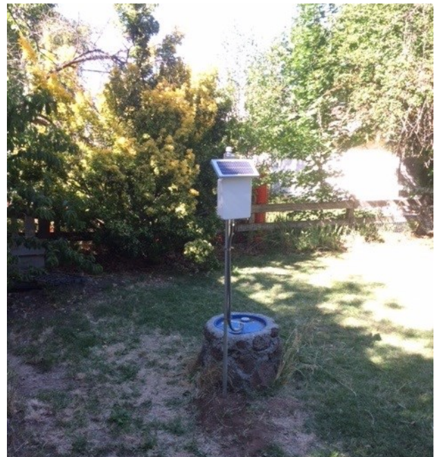
Groundwater well elevation logging equipment on a private landowner's property
